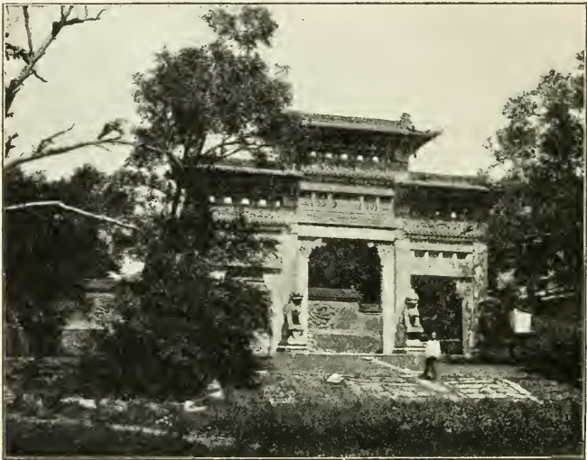
The entrance gate to North Mausoleum, Mukden
