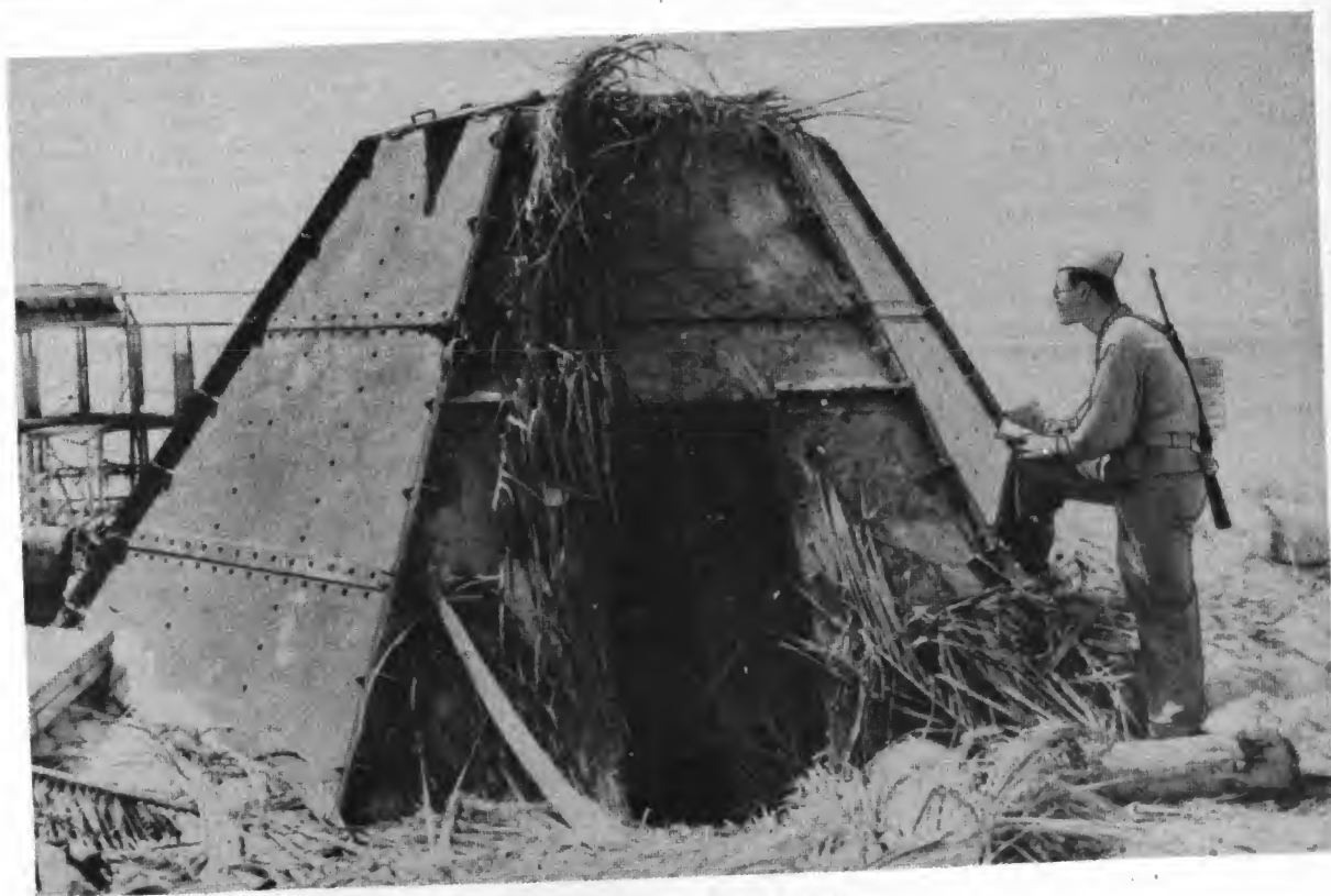
Figure 145. A hexagonal steel pillbox.
