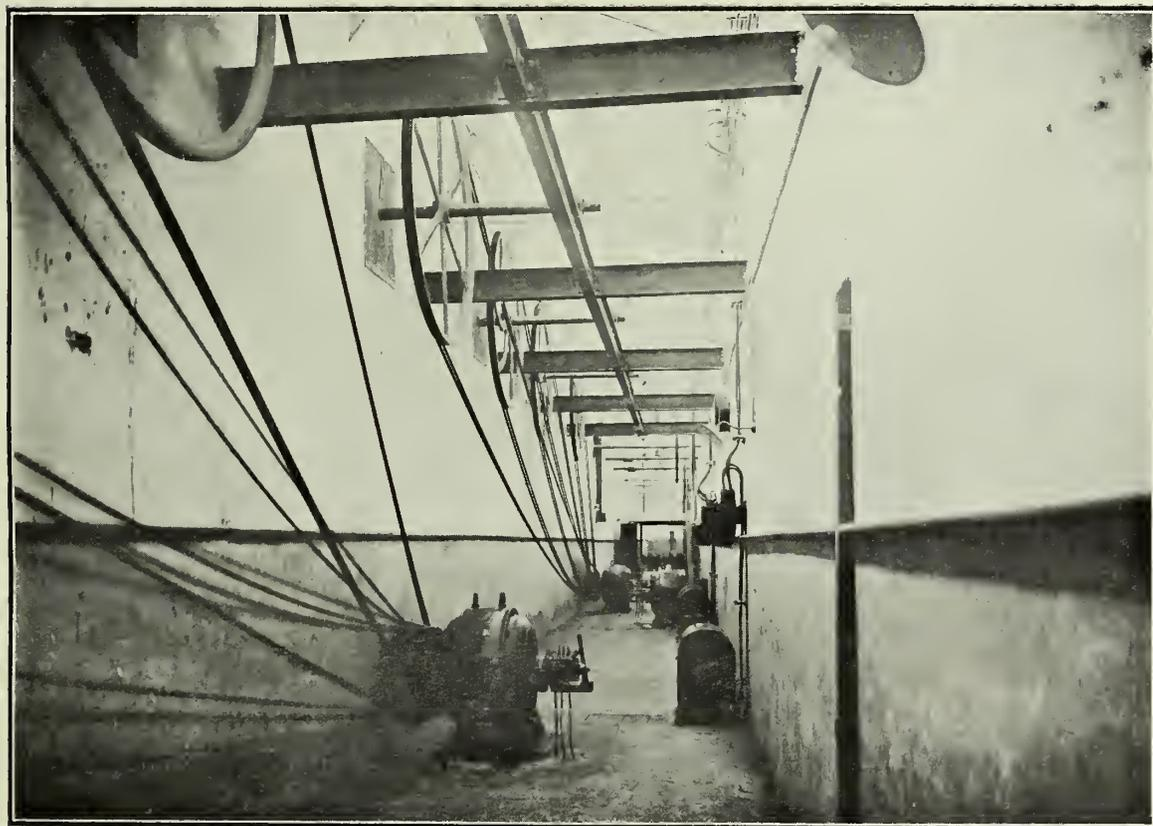
A local installation of five 80 horse power motors driving 1,000 looms.
