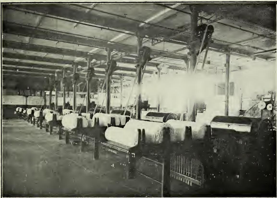
A local installation of nine  $7\frac{1}{2}$  horse power motors driving cotton scutching machines.
