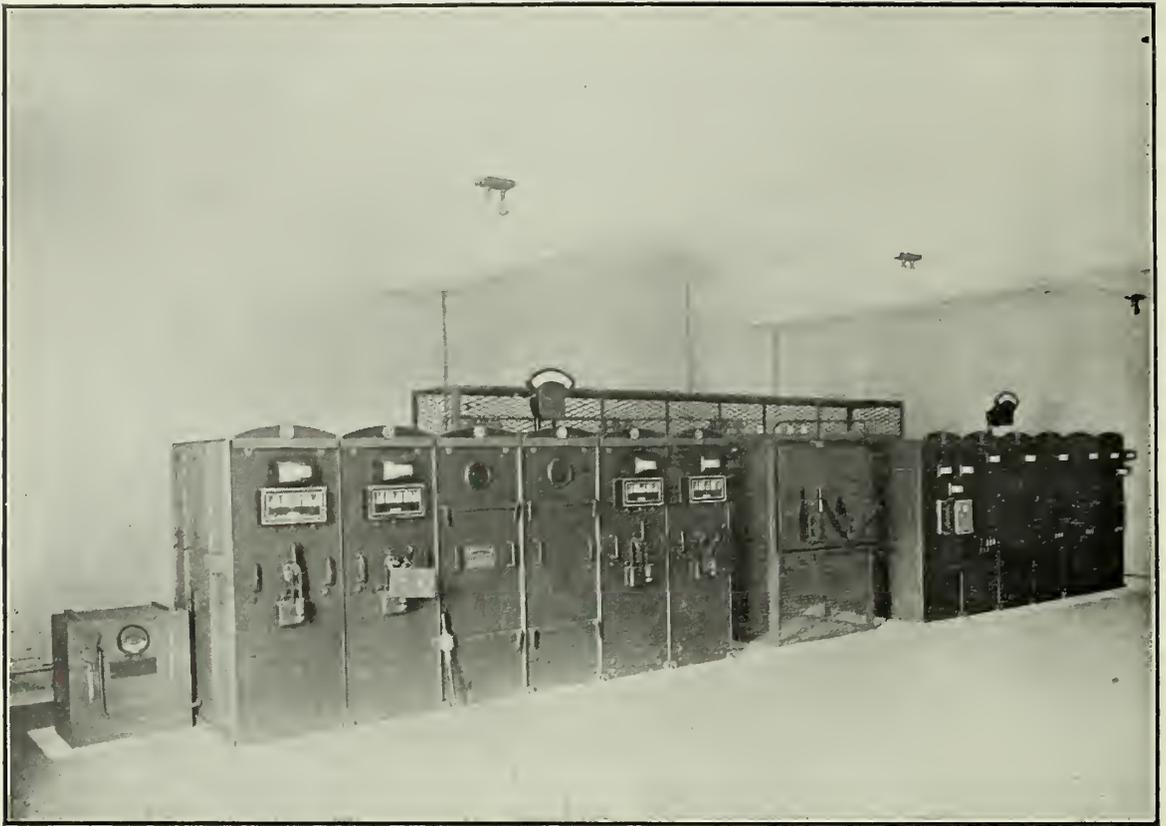
Three-phase 2,000 kilowatt sub-station. Interior—Extra High Pressure Switch Gear.
